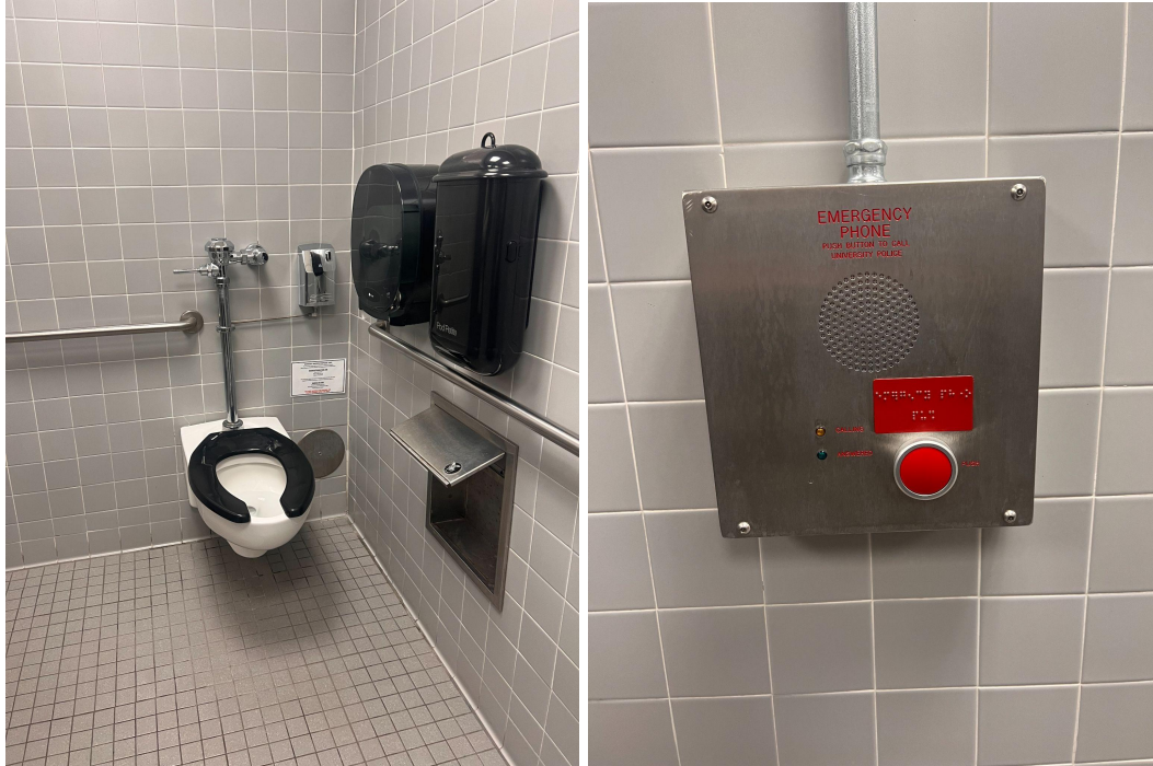
Image Description: (Left) Toilet placed between two pull bars on either side. To the right of the toilet a toilet paper dispenser, and trash bin are propped above the pull bar. The walls and floors are tiled. (Right) Emergency phone and button hung onto a tiled wall.
