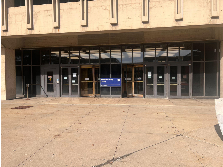
Image Description: Six entrances in total, two sets of doors on either side of two revolving doors. The door furthest to the right is the accessible door with the accessible push button. The concrete ground is textured and cracked.
